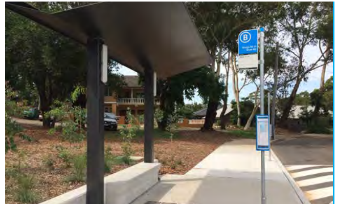
Bus stop with shelter canopy, seating, and signage
