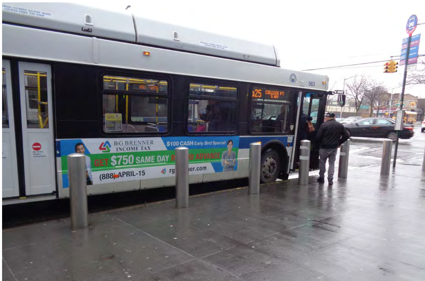
Well-protected boarding area with bollards
