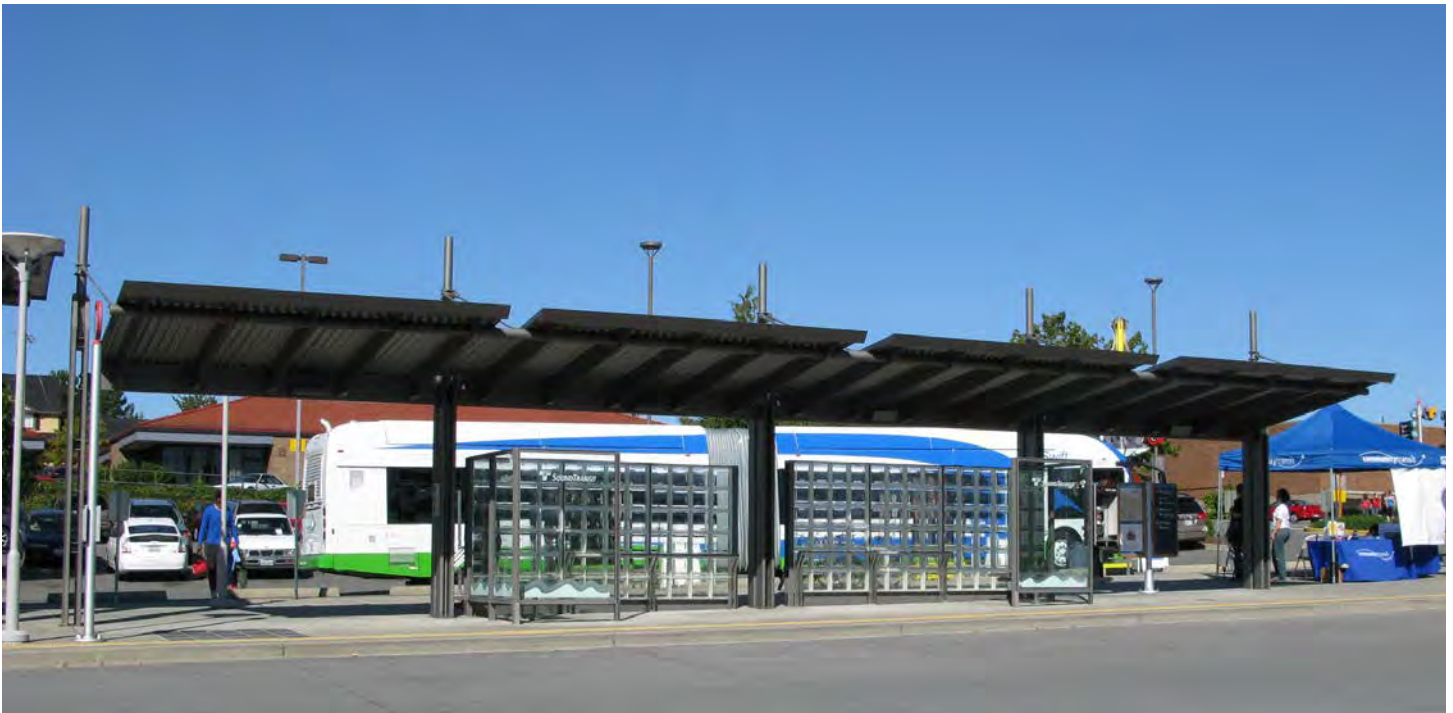
Canopy shelter utilizing durable materials
