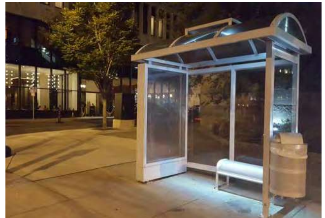
Bus stop lighting
